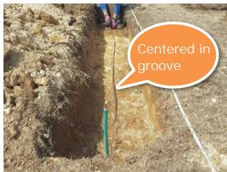
① Drill trenches and lay grounding wires
