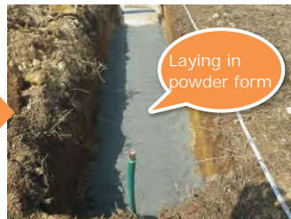
② Laying BIO SAN-EARTH (1 bag: 3m)
